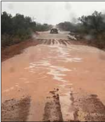
Taking a submerged road in the North West during rain.
